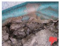
Not buried deep enough & ground poorly compacted.
