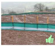
Bottom buried up to red line & backfill firmly compacted.
